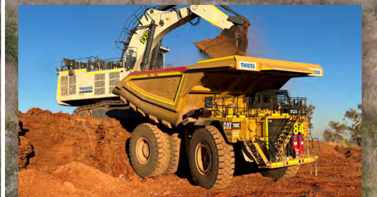
Thiess secured contract with Groote Eylandt Mining Company (GEMCO) Southern Lease manganese project, re-entering the Northern Territory
